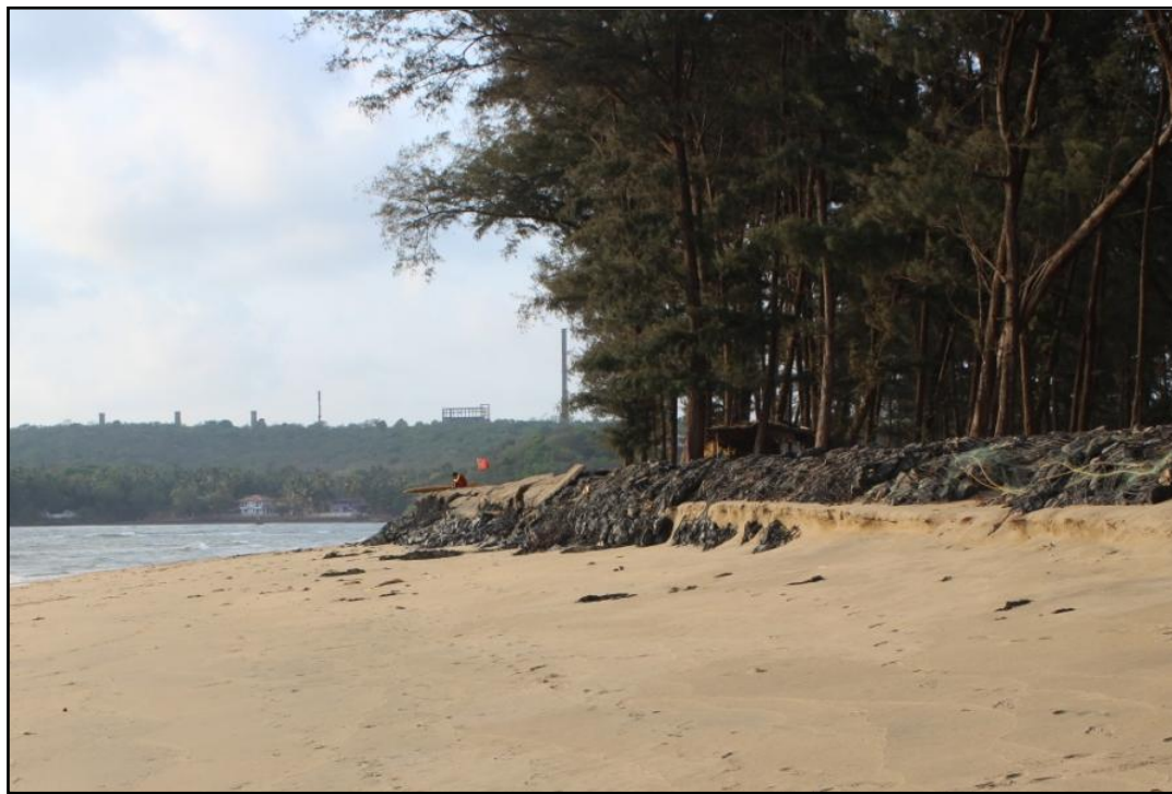
Plate 46: Severe erosion at Keri (46E10NE)
