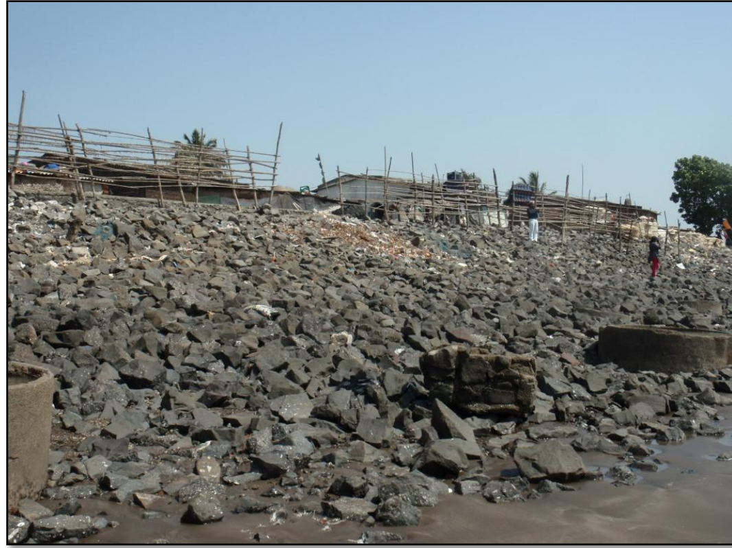
Plate 18: Seawall at Dahanu (47A09NE)
