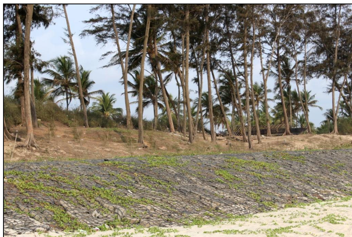
Plate No.59: Sea wall at Betalbatim (48E15SE)
