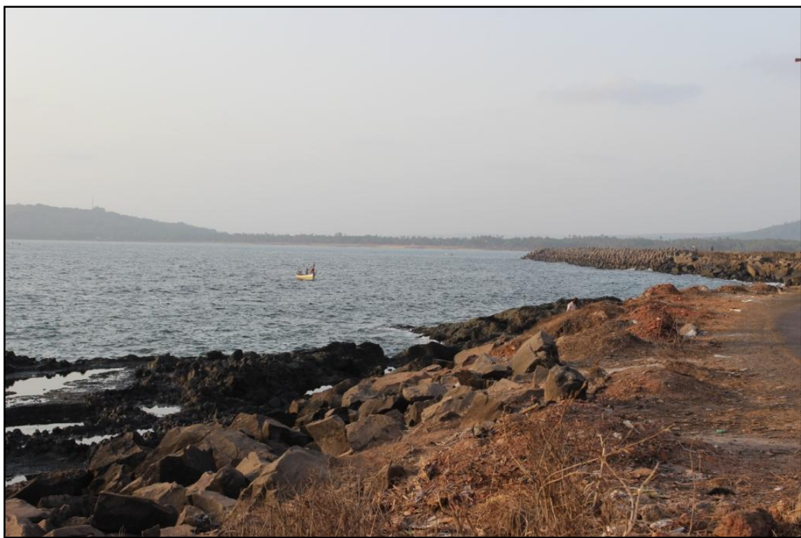
Plate 37: Protection measures near Mirya Bandar (47G08SW)
