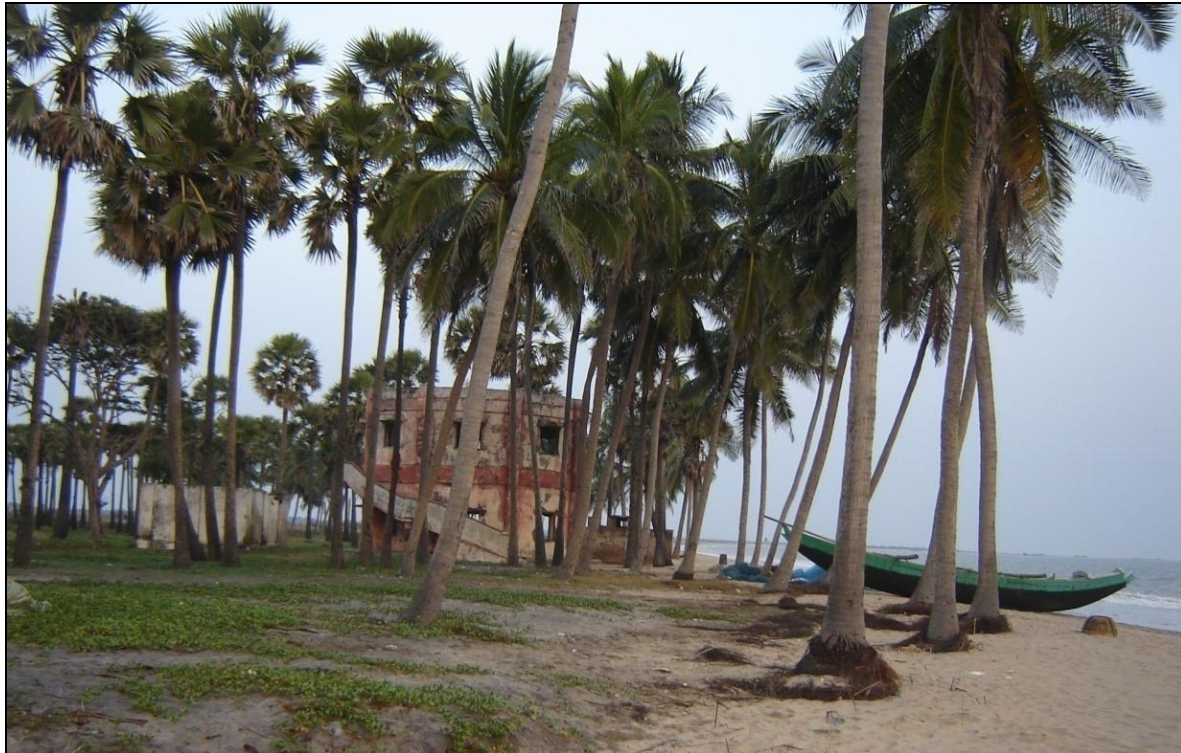
Plate 37: Severe erosion, west of Vasishta Godavari river mouth, coconut tree plantation uprooted (65H11SE)
