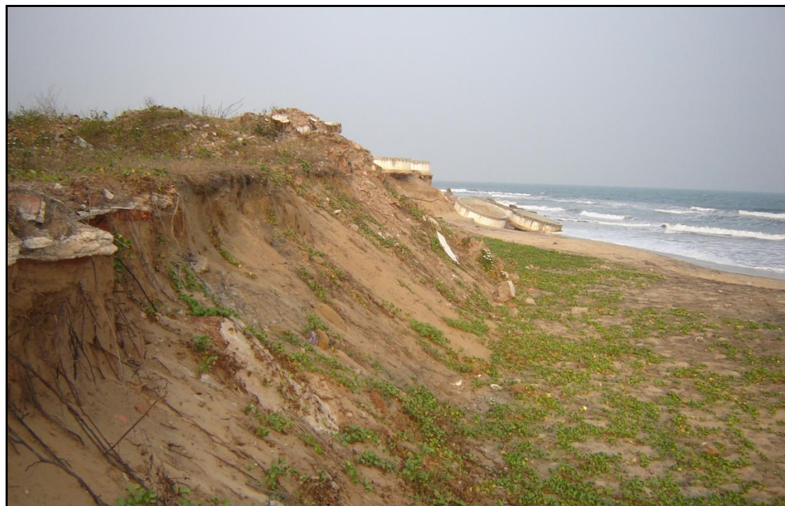
Plate 24: Hatcheries destroyed due to coastal erosion near Shamvanipakalu (65K08SE)
