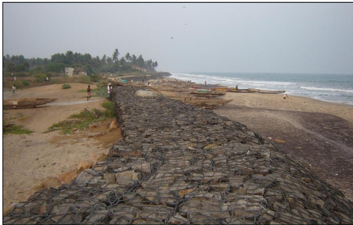
Plate 29: Sea wall constructed near Uppada (65K08SW)
