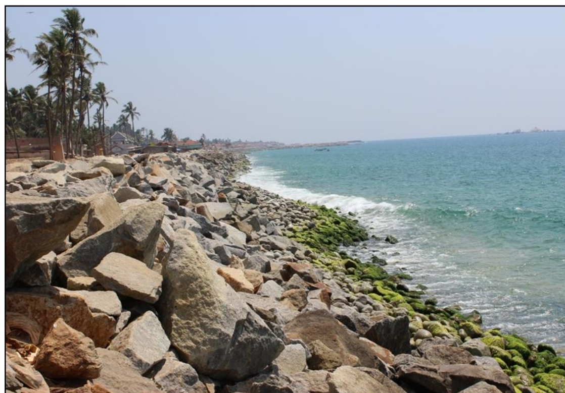
Plate 75: Severe erosion along roadside NW of Melmidalam, Kanniyakumari district (58H04NE)
