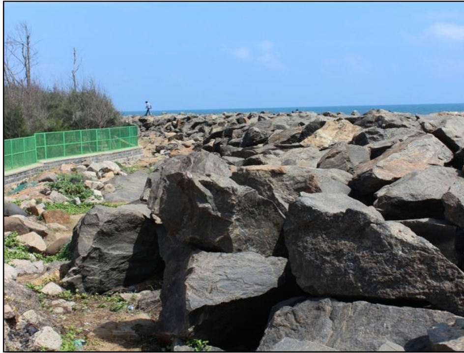
Plate 49: Sea wall at Mahabalipuram shore temple, Mammalapuram, Kancheepuram district (66D02SE)
