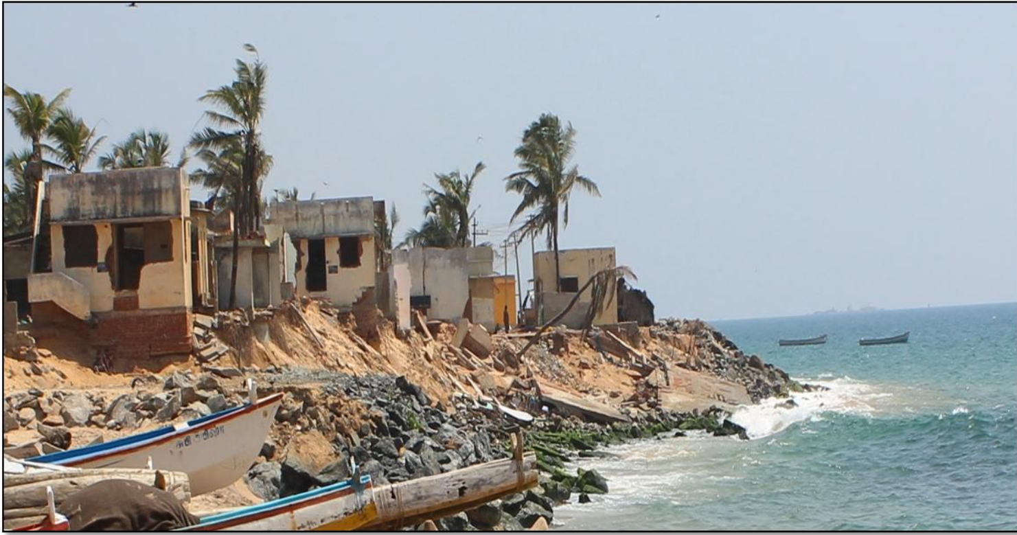
Plate 76: Severe erosion at Puttantura, Kanniyakumari district (58H04NE)
