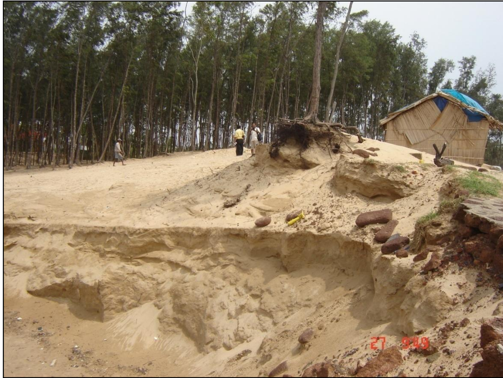
Plate 64: Erosion at Digha (73O10SW), SW parts of West Bengal coast
