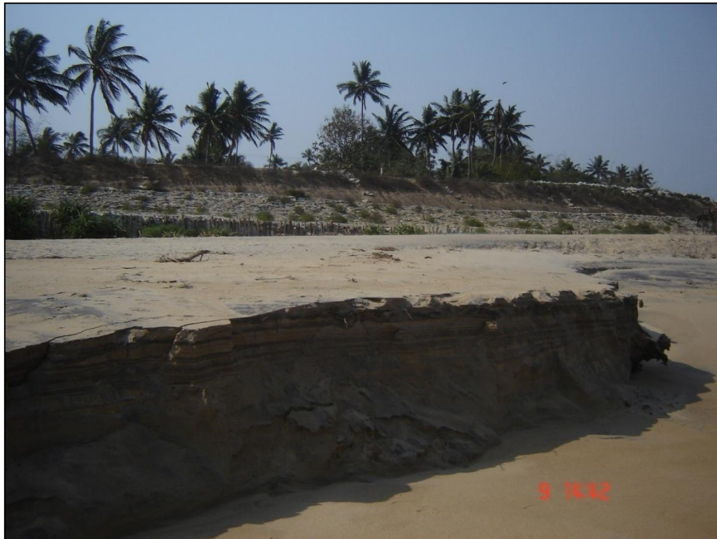
Plate 38: Severe erosion at Pentha (73L14SW) along central parts of Odisha coast
