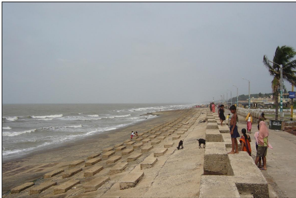
Plate 59: Protection structure at Digha(73O10SW), SW parts of West Bengal coast
