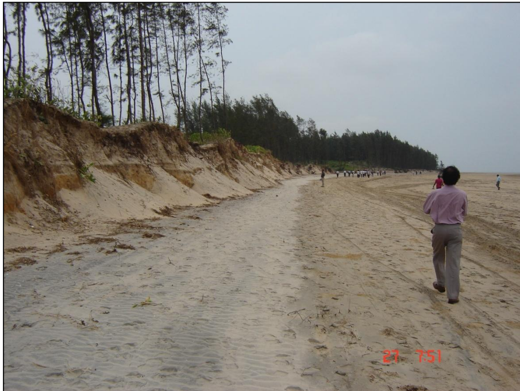
Plate 56: Erosion along eastern parts of the Subarnarekha estuary (73O06SW), Odisha coast
