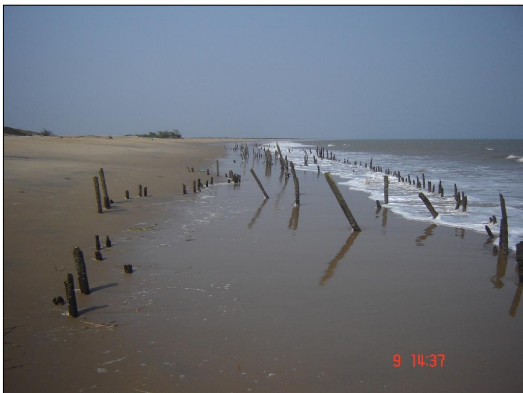
Plate 39: Protection measures wiped off by Sea at Pentha (73L14SW) along central parts of Odisha coast
