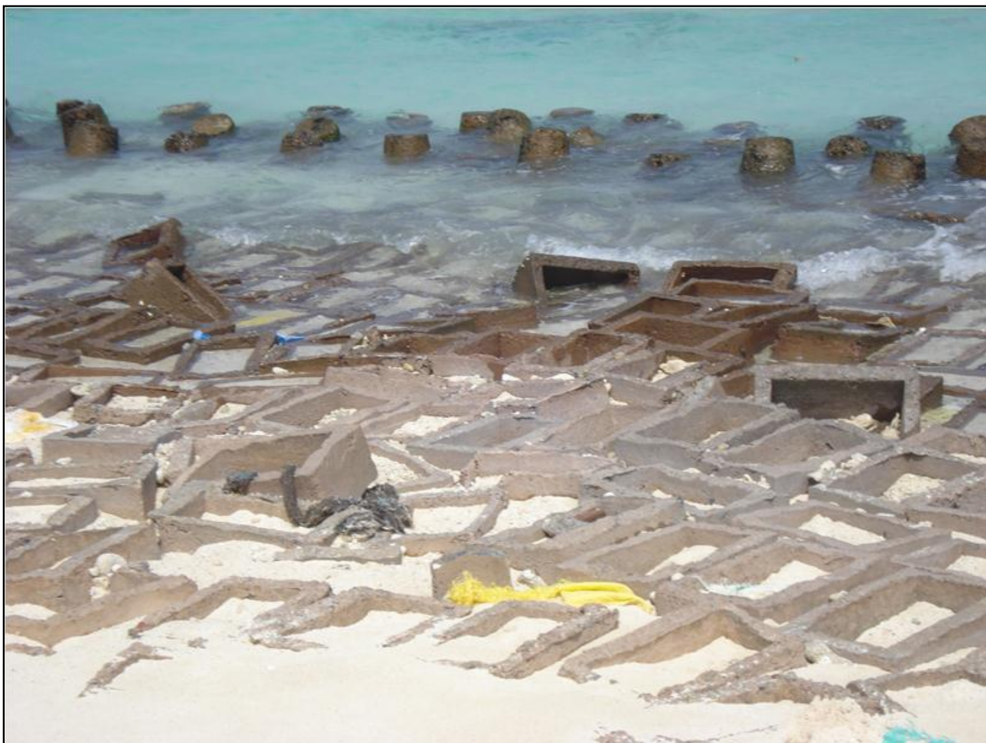
Plate No. 12: Hollow Block for protection near Puthiyapally, Kavaratti, Lakshadweep
