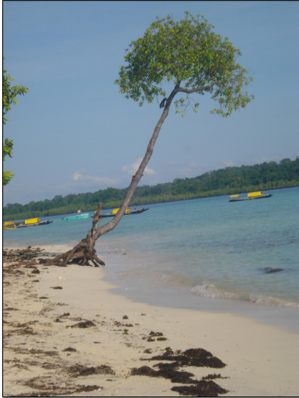
Plate No. 15: Erosion at Havelock island
