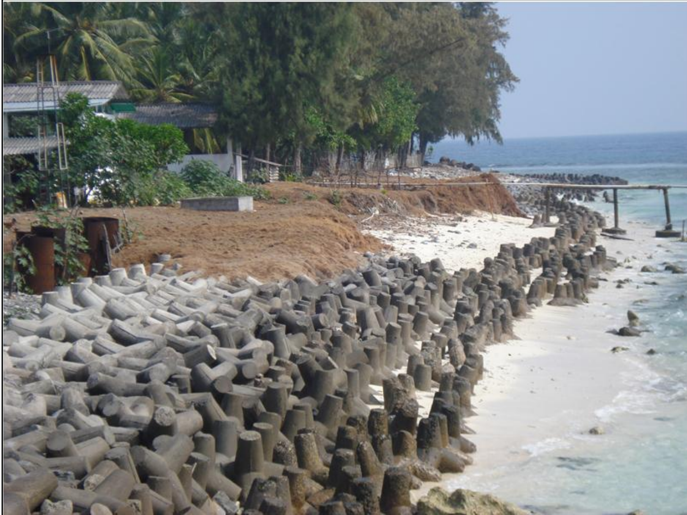
Plate No. 11: Beach Protection near Kavaratti Harbour, Lakshadweep
